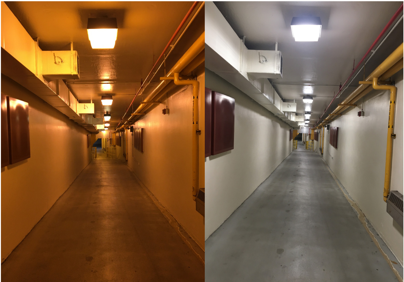
The MWRD is working to become more sustainable by pursuing an array of environmental improvement projects, like LED lighting, while also developing technologies for renewable energy generation. LED light upgrades improve a pedway at the MWRD's Stickney WRP and can produce light up to 90 percent more efficiently than incandescent light bulbs.
