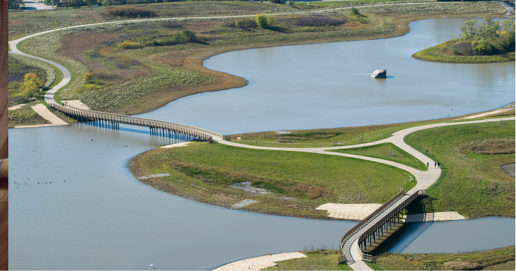
The Buffalo Creek Reservoir Expansion Project will alleviate flooding for downstream communities while improving public recreation spaces at Buffalo Creek in the Lake County Forest Preserves.
