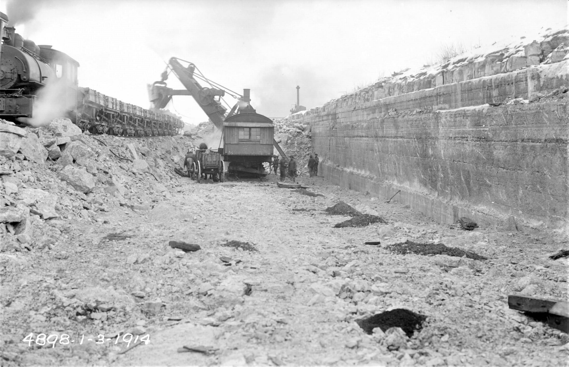
Rock excavation near the west end of the Calumet-Sag Channel, January 1914
