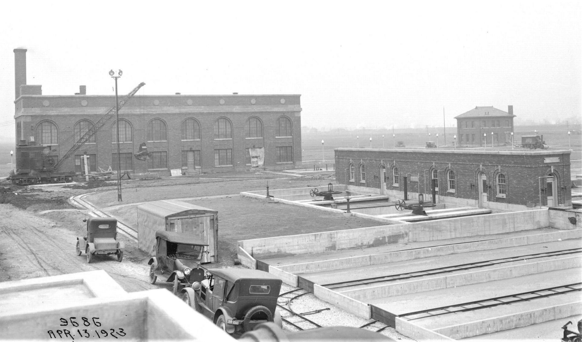
Calumet Plant, experimental activated sludge process unit, April 1923
