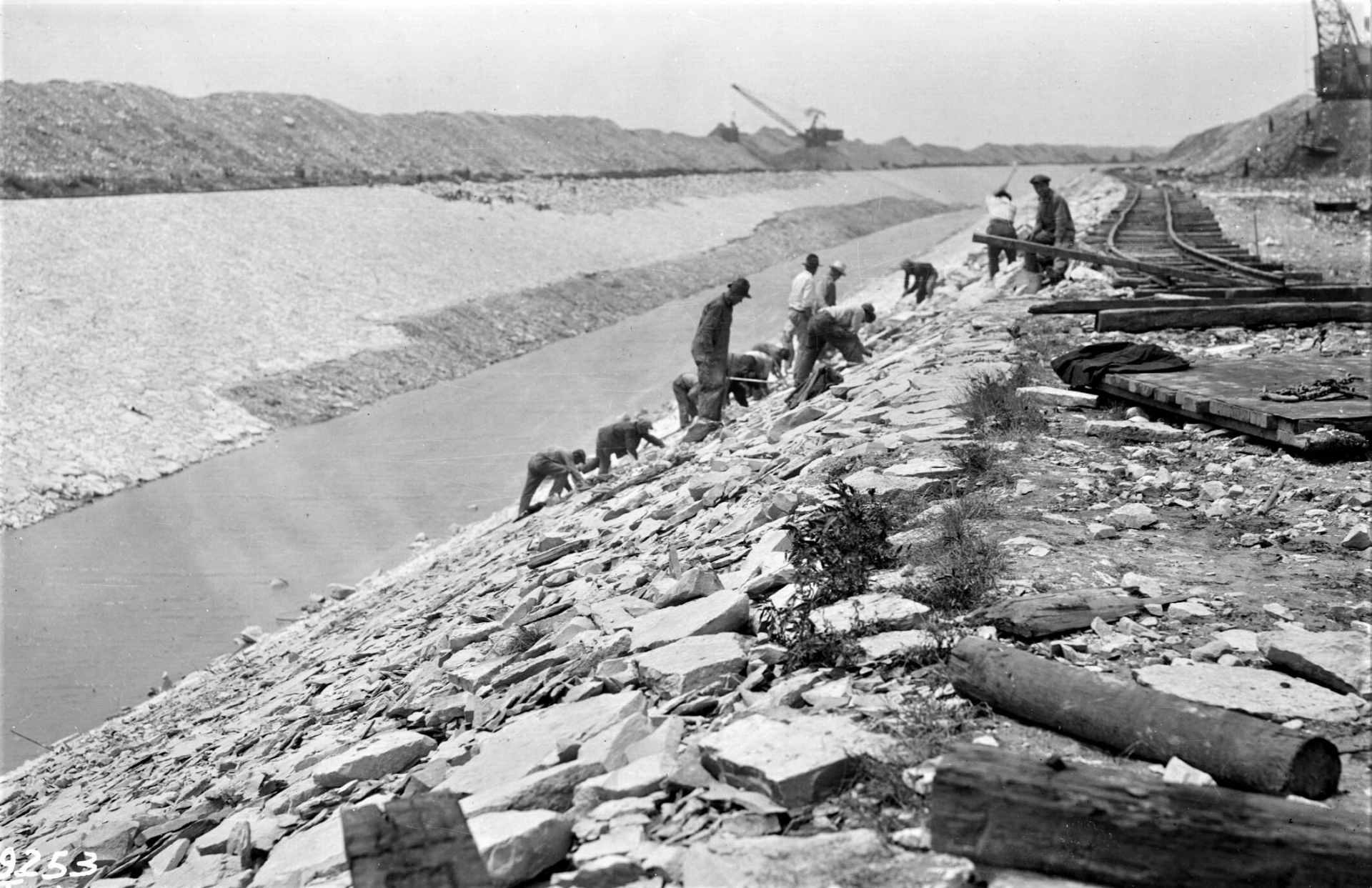
9253 Hand placing rock riprap after side slope failure, looking southwest near Pulaski Road, July 1922
