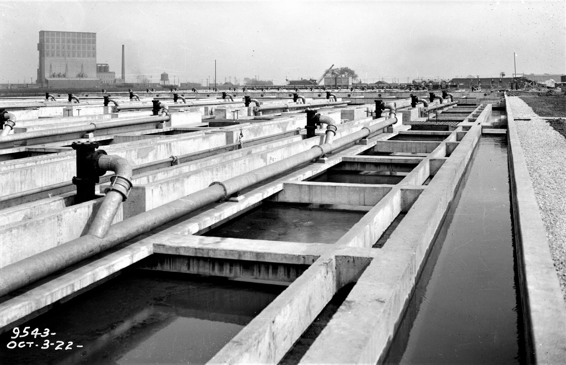
Calumet Plant, Imhoff tanks in operation, October 1922
