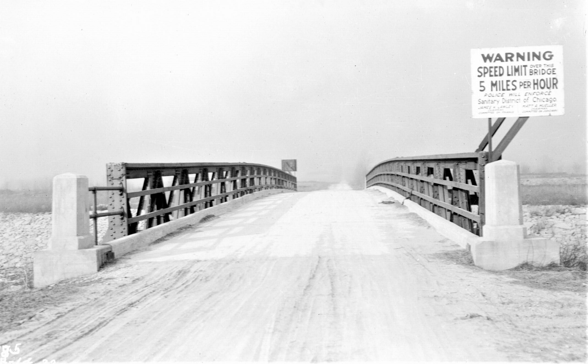
Looking north across Piper Road (Ridgeland Avenue) bridge, February 1922
