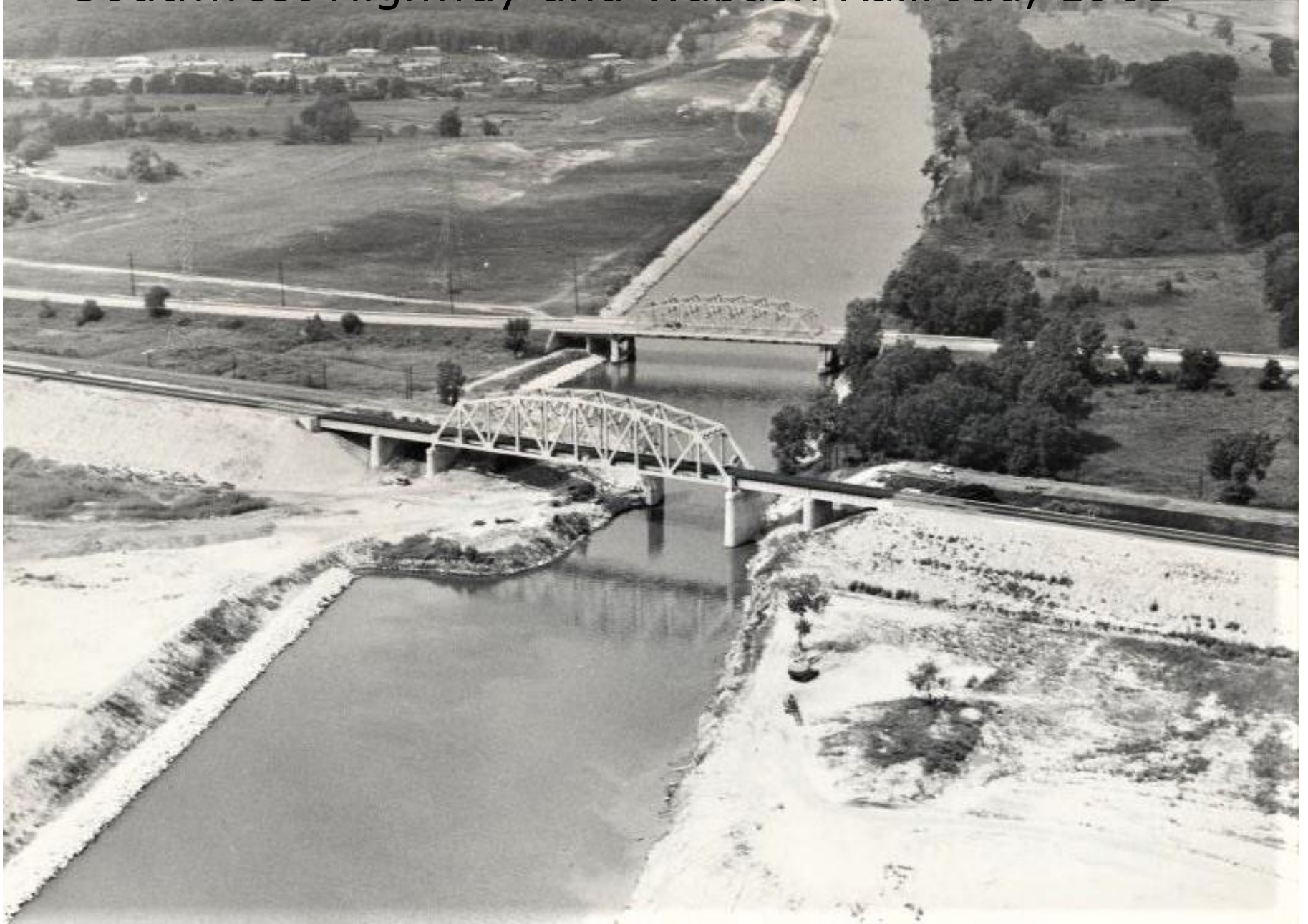
Looking west widening the Calumet-Sag Channel, Southwest Highway and Wabash Railroad, 1961
