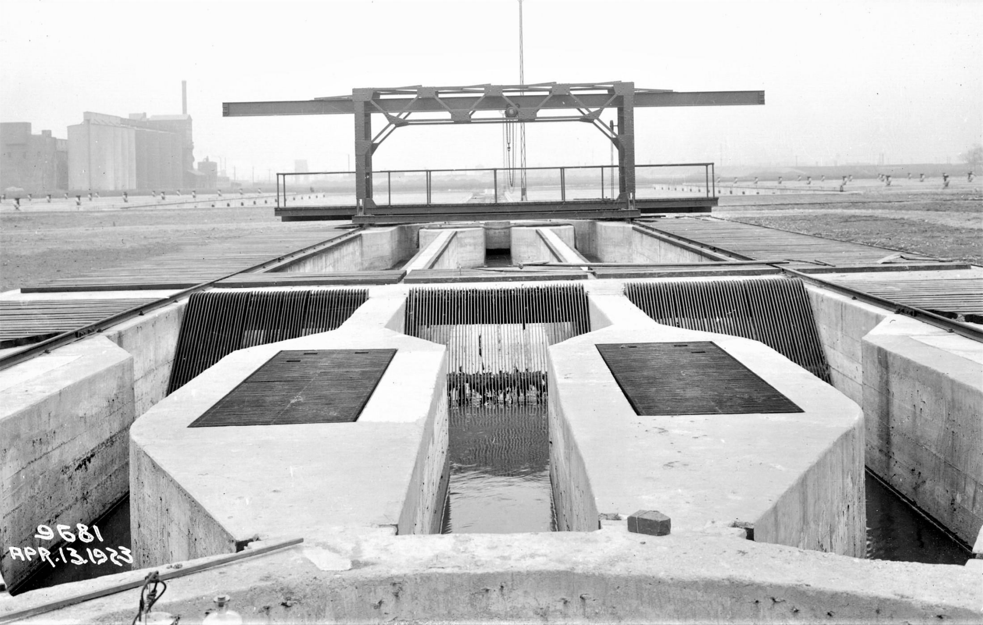
Calumet Plant, raw sewage screens and grit tanks, April 1923
