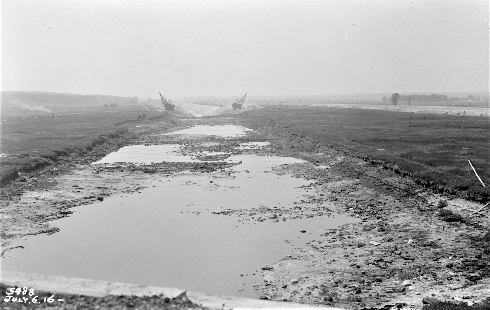
Looking east from the Wabash Railroad after hydraulic dredges removed marsh, July 1916
