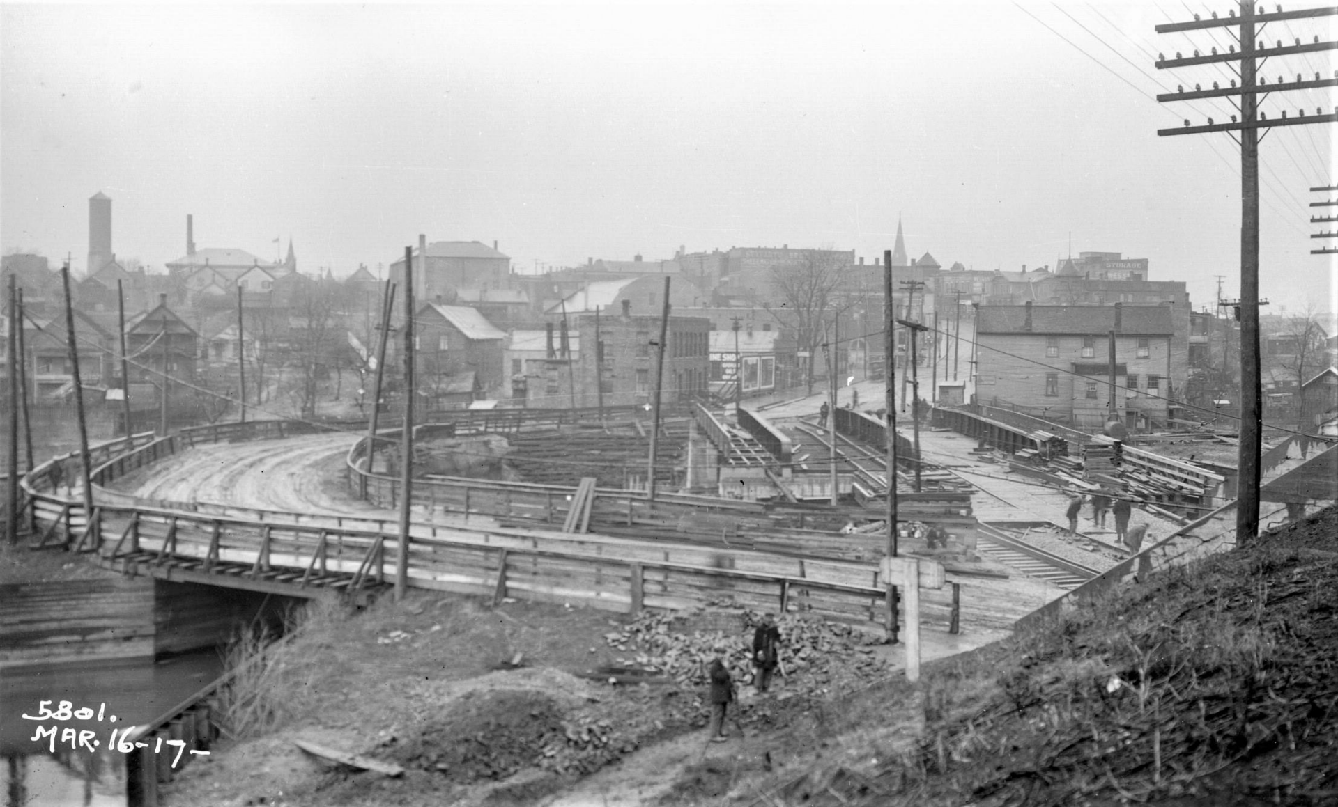
Looking north at Western Avenue temporary and permanent bridge construction, March 1917
