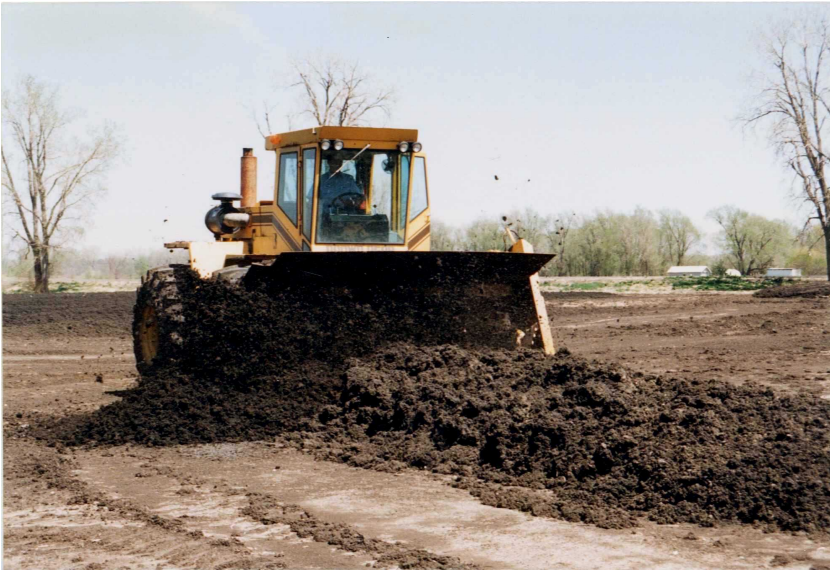
biosolids composting, Topeka, KS
