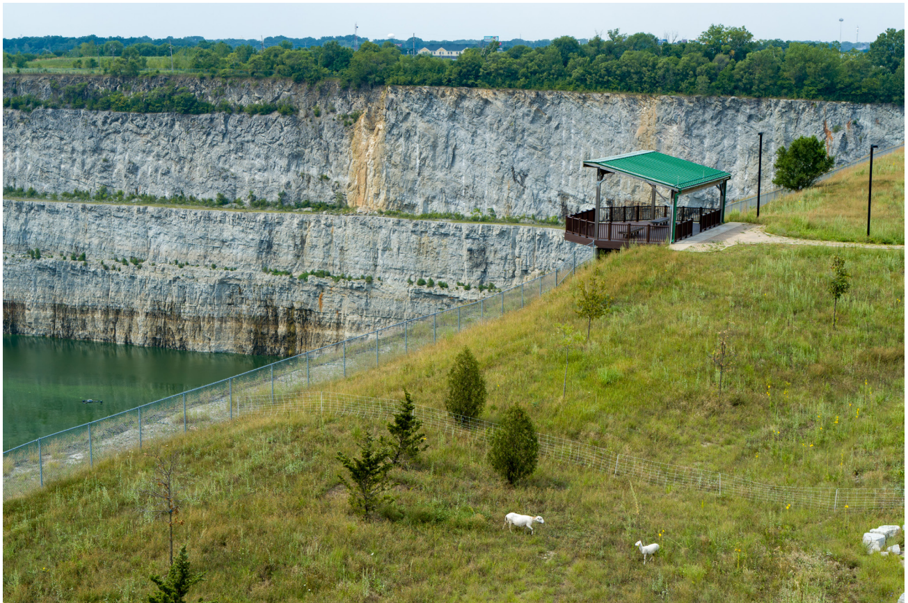
The Thornton Composite Reservoir provides 7.9 billion gallons of storage. Since becoming operational in 2015, this reservoir has prevented more than 53.4 billion gallons of combined sewage from entering the area waterways.
