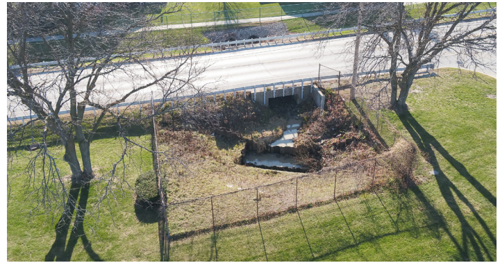
The existing junction structure near the Nathan Hale School will be replaced to improve conveyance of stormwater from the new 135th St. storm sewer to the Crestwood Drainage Ditch.
