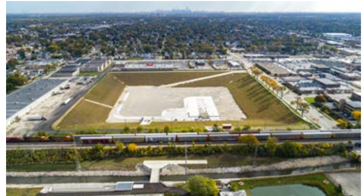
The Addison Creek Reservoir provides 195 million gallons of storage capacity and connects with the Addison Creek Channel (at bottom). Photo taken October 2022.
