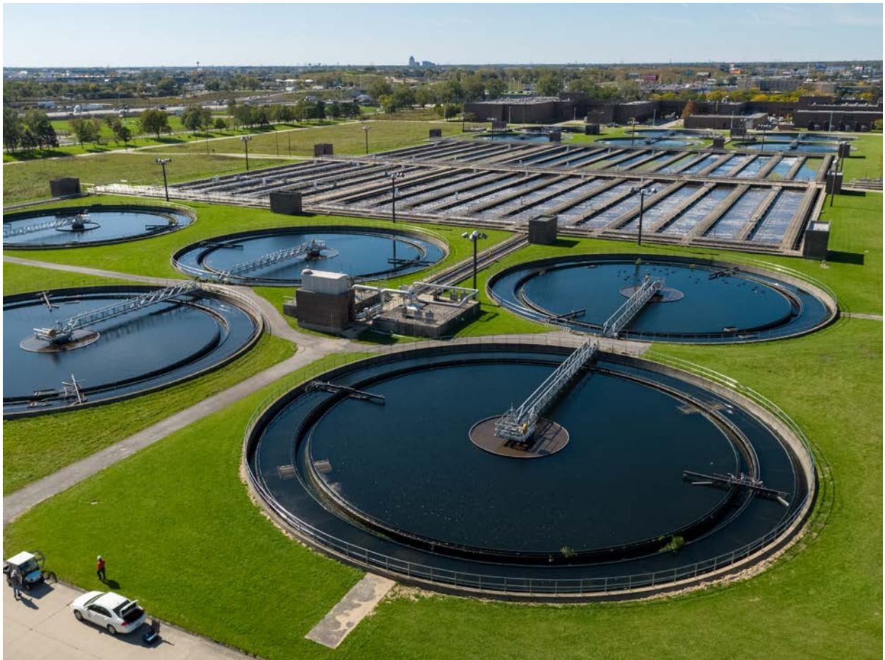
The Kirie Water Reclamation Plant in October.
