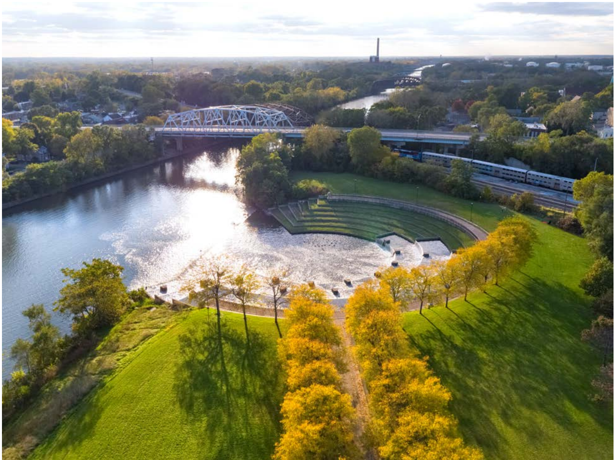
Autumn colors at the MWRD's Sidestream Elevated Pool Aeration (SEPA) station in Blue Island on October 17. The SEPA station is number three of five, all of which are located on the Cal Sag Channel and function to improve water quality by adding oxygen to water via manmade waterfalls.
