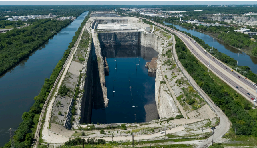
The McCook Reservoir, the last component of the Tunnel and Reservoir Plan system, serves 3.1 million people in 37 communities.
