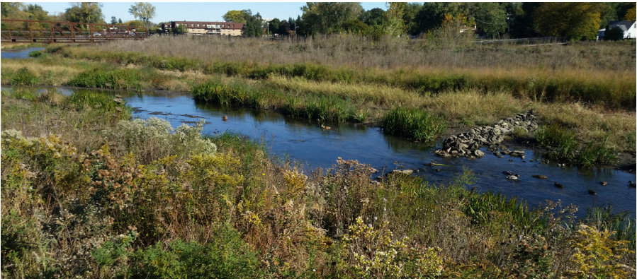
Buffalo Creek was improved by the District under the Heritage Park Flood Control Facility project. Other improvements featured on the project included widening of the creek banks, new stormwater storage areas within Heritage Park, and recreation amenities planned in coordination with the Wheeling Park District.
