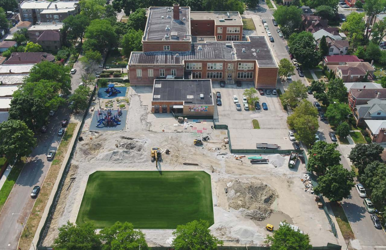
▲ Construction of the Space to Grow schoolyard at Boone Elementary School.
