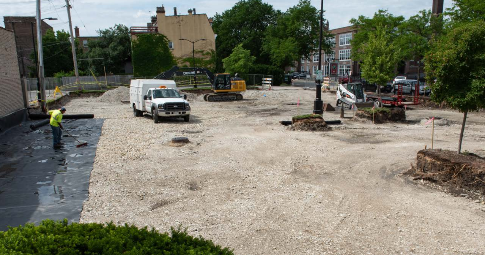
▲ Installation of permeable pavement in La Grange.
