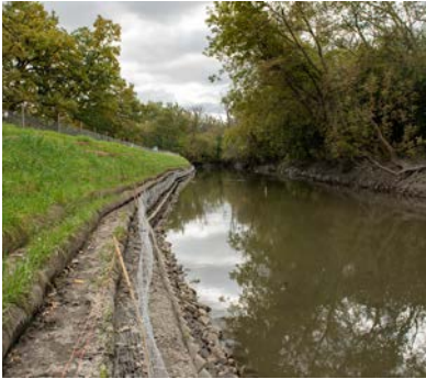
▲ Streambank stabilization on Addison Creek.
