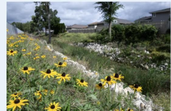
Channel improvements along the Crestwood Drainage Ditch
