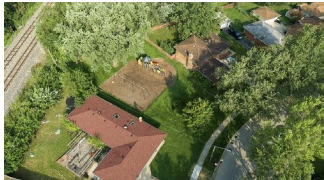
The North Creek Flood Relief Project, funded by the District at a cost of $1.6 million, involved constructing a new culvert for North Creek to alleviate flooding and safeguard 56 residential structures in the vicinity of Flanagin Park.
