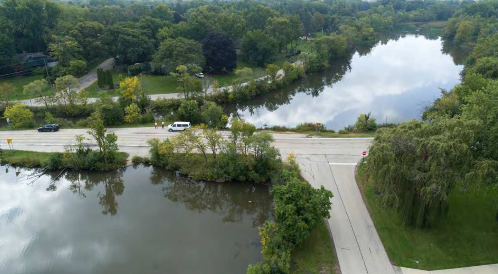
The Willow Road Flood Control Project is designed to provide relief for Prospect Heights residents who have not been able to enter or exit their homes on rainy days.
