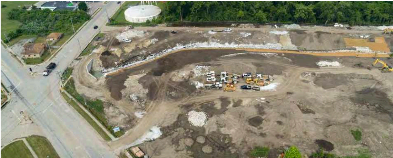
Excavation and construction at the Phase 1 area for the Robbins Heritage Park and Midlothian Creek Restoration Project.
