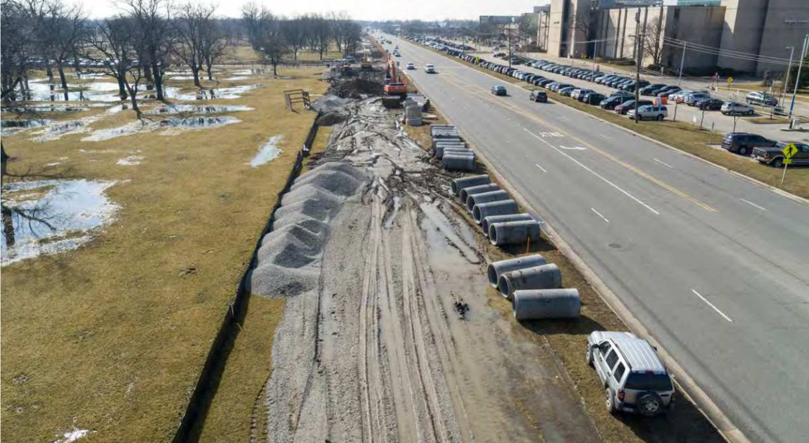
A view to the south shows excavation and placement of pipe during construction along 1st Avenue near Miller Meadow Nature Preserve in Forest Park.
