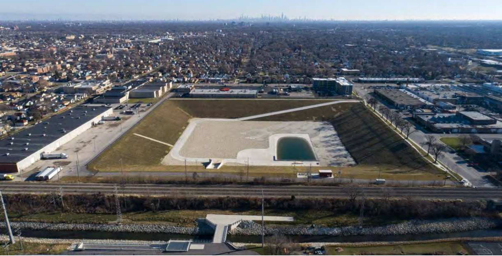
A view to the east shows the Addison Creek Reservoir in Bellwood on Dec. 12, 2023. The Addison Creek Reservoir and the Addison Creek Channel Improvements are two connected flood control projects that will work together to significantly benefit communities along Addison Creek, including Bellwood, Northlake, Stone Park, Melrose Park, Westchester and Broadview. The 600-acre-foot Addison Creek Reservoir will hold 195 million gallons of storage capacity and connect with the Addison Creek Channel to protect the communities from overbank flooding.
