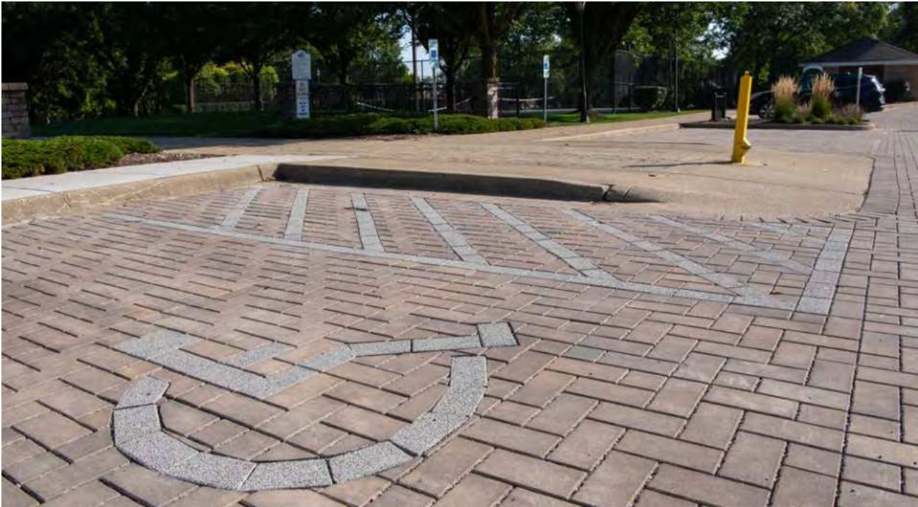
Permeable pavers were used to replace two parking lots in Countryside at Countryside Park.
