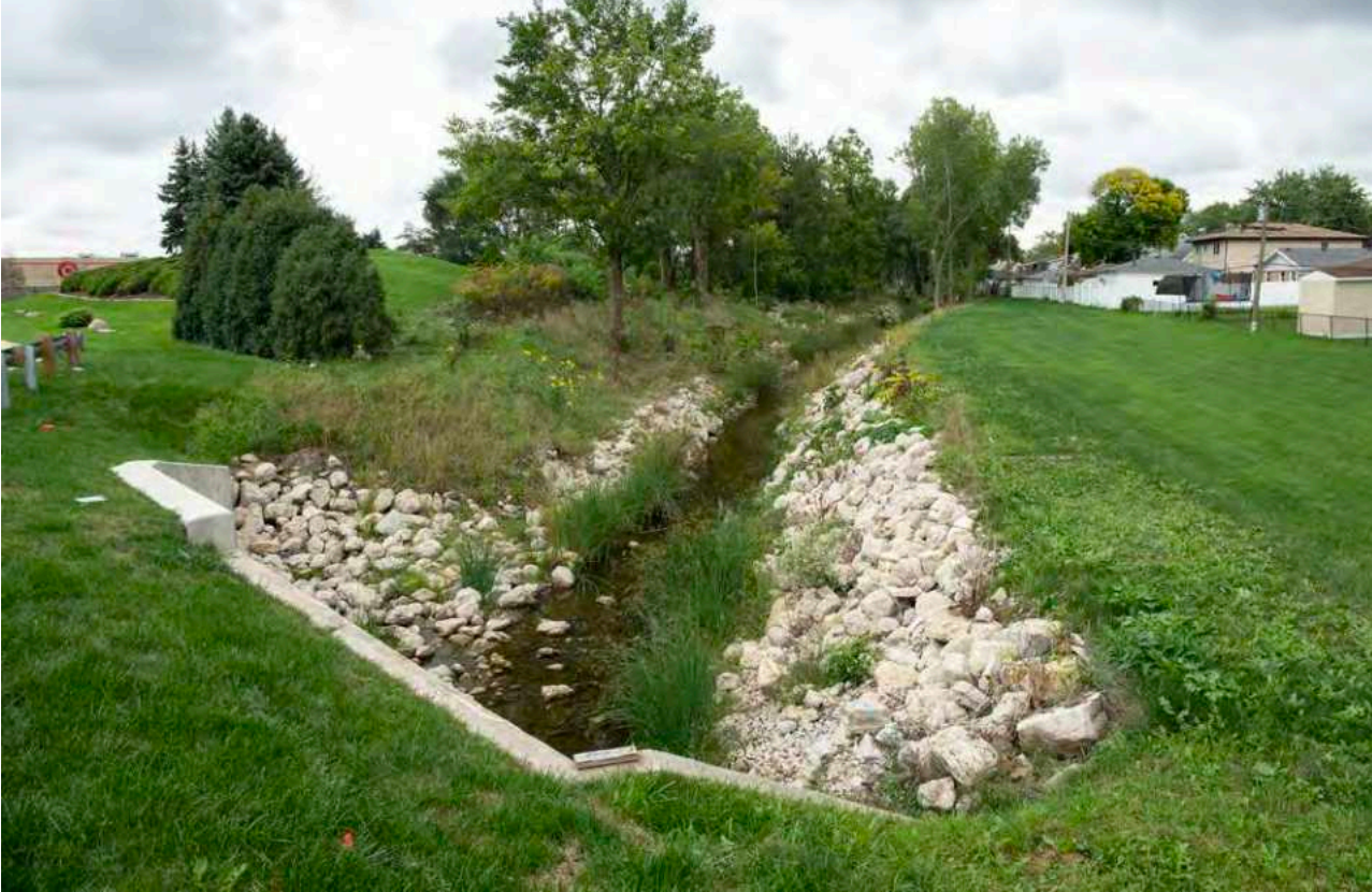
A view looking south from the new culvert under Cal-Sag Road in Crestwood, showing the improved Crestwood Drainage Ditch.
