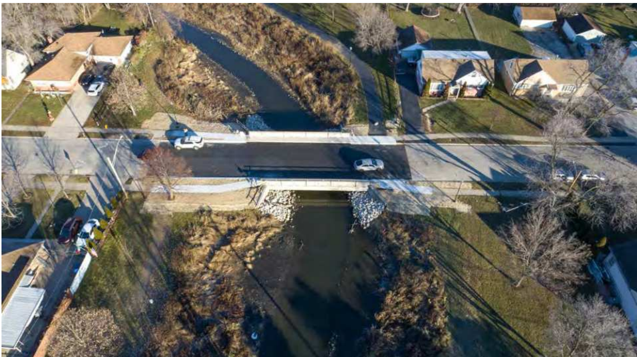
Addison Creek Channel project is designed to improve channel conveyance through six municipalities.
