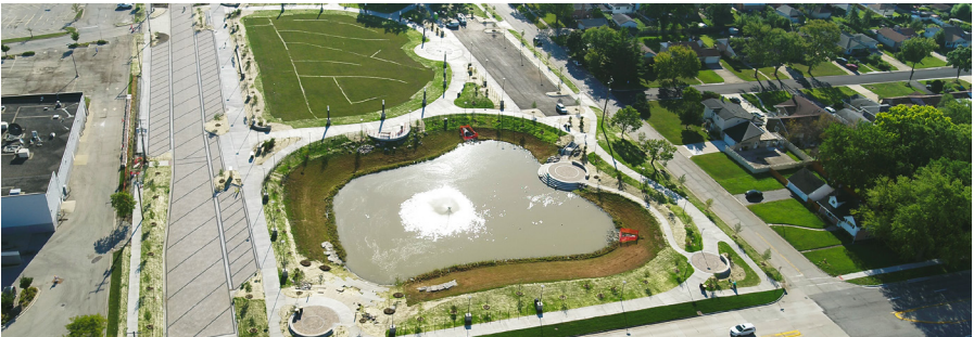
The Golf Mill Park stormwater project in the Village of Niles utilizes green infrastructure elements and permeable pavement to mitigate flooding and to improve local water quality.
