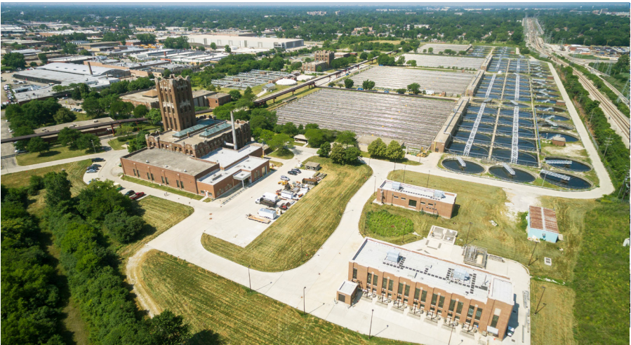
The O'Brien Water Reclamation Plant serves over 1.3 million people in communities north of downtown Chicago and features the largest ultraviolet disinfection facility for a wastewater plant in the United States, with a capacity to treat over 450 million gallons per day.
