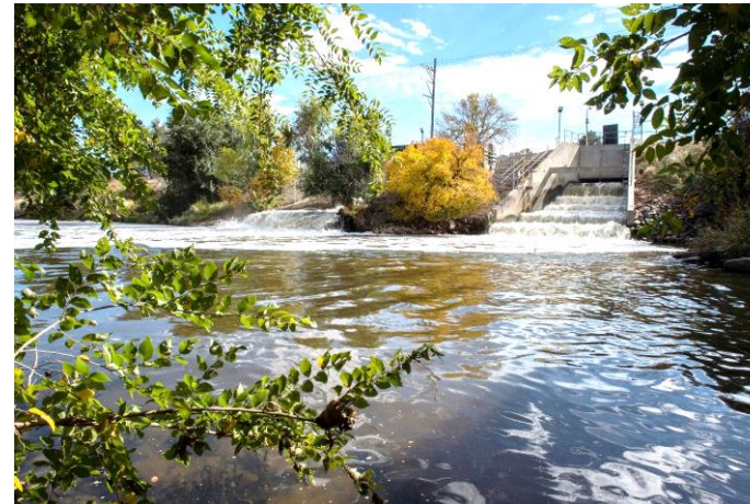
South Platte River at Outfalls
