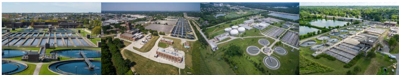
Kirie, O'Brien, Egan, and Hanover Park WRPs are four of seven wastewater treatment facilities that comprise the North Service Area with regulatory permit requirements for phosphorus limits coming online in the new future.
