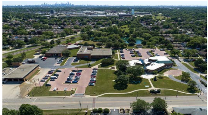
Six new green parking lots using permeable pavers to collect more stormwater and reduce the load on local sewers and waterways can be seen at North Riverside Commons complex.
