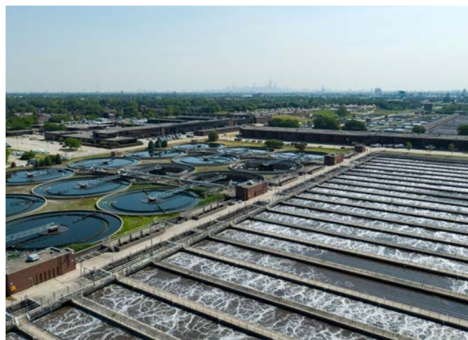
The Stickney Water Reclamation Plant (WRP) is one of the largest wastewater treatment facilities in the world. It serves residents in the central part of Chicago and 46 other communities within a 260-square-mile area. The Stickney WRP consists of two plants: the original West Side Plant, which was placed in service in 1930, and the Southwest Plant, which was placed in service in 1939.
