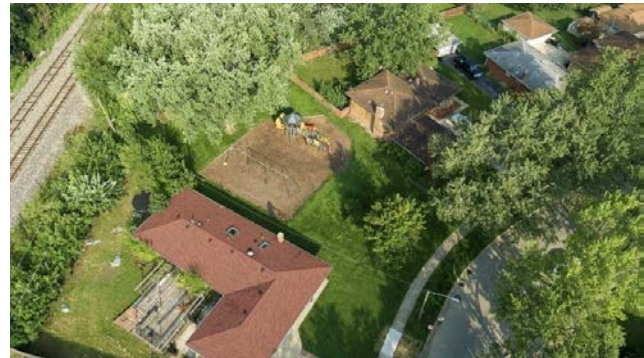
The North Creek Flood Relief Project, funded by the District at a cost of $1.6 million, involved constructing a new culvert for North Creek to alleviate flooding and safeguard 56 residential structures in the vicinity of Flanagan Park.
