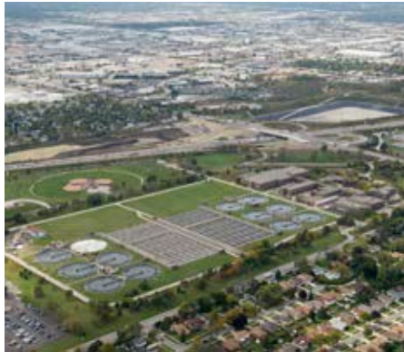
Kirie Water Reclamation Plant
