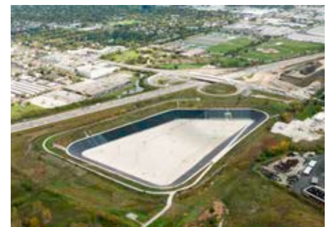
The Majewski Reservoir, part of the MWRD's Tunnel and Reservoir Plan (TARP), provides 343 million gallons of combined sewage storage for communities in the Kirie WRP service area.
